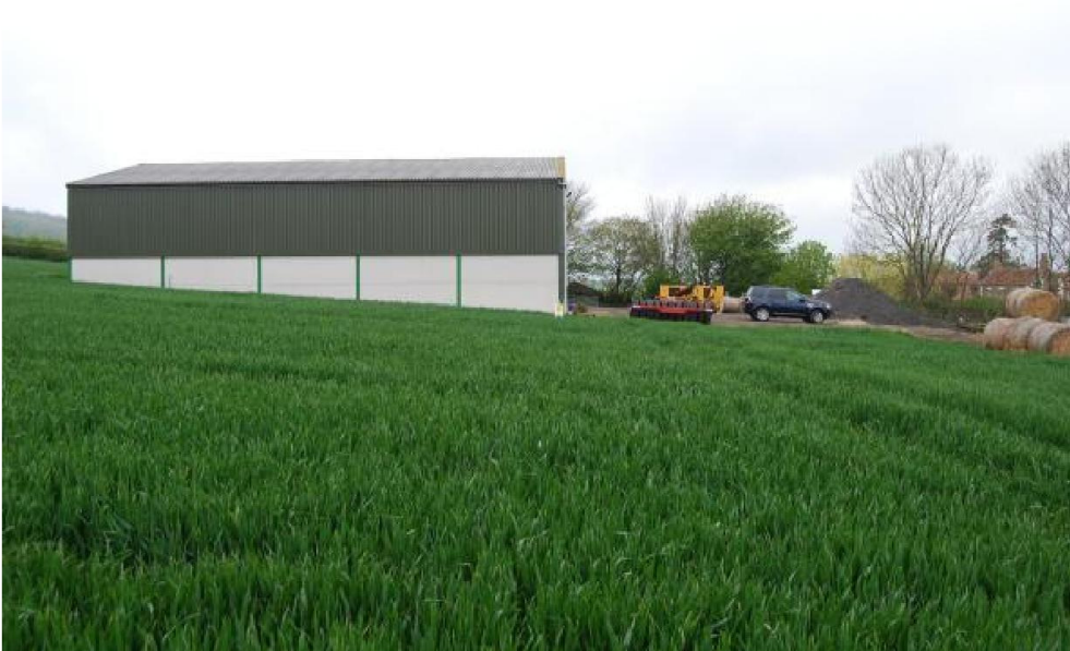
View across site to west.
