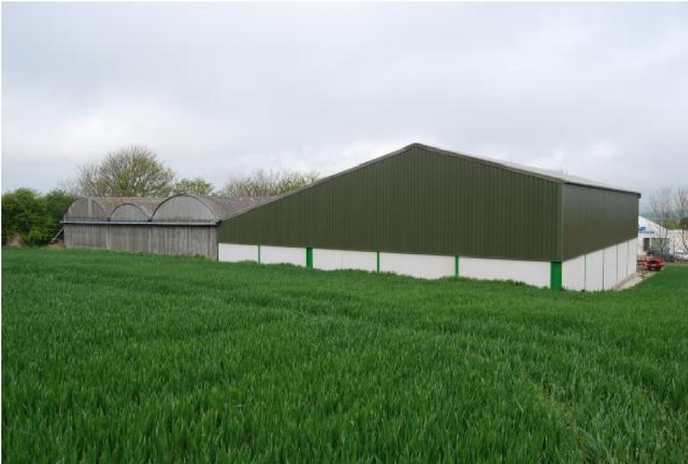
Adjacent buildings view to north west.
